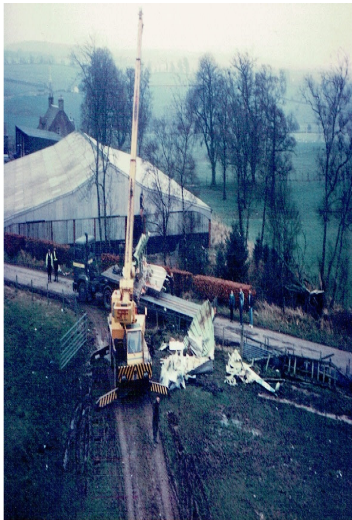
Above: Lifting wreckage onto a trailer.
